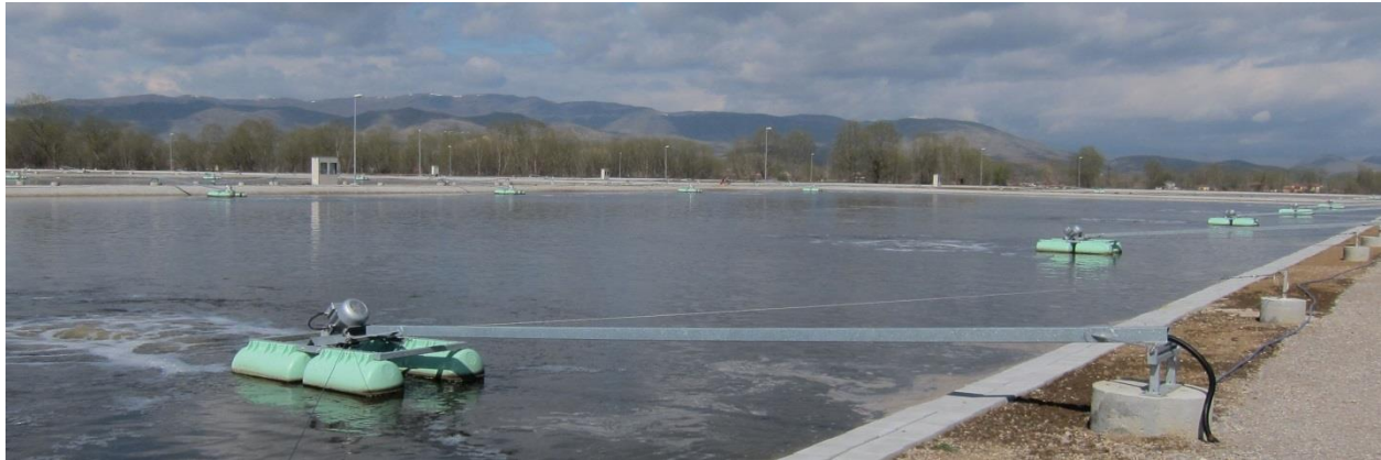
WWTP Korça – Aerated Lagoon System
