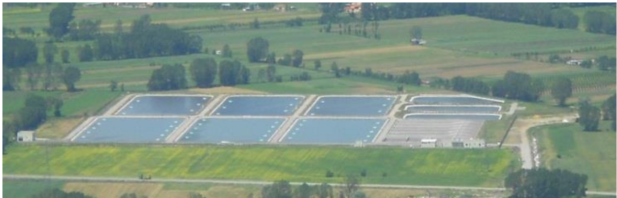
WWTP Korça – Aerated Lagoon System
