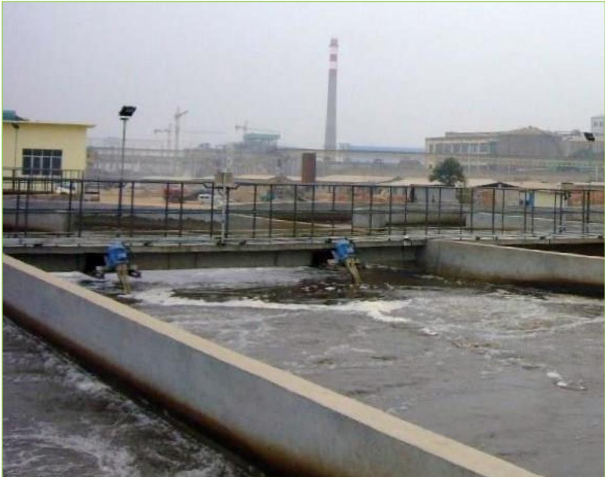
At the end of 2007 the carrousel shaped oxidation ditch of Funan sugar mill was equipped with 34 sets of OxyStar Aerators OS 30.0 (22.0 kW each). The aeration tank has a total volume of approx. 35,100 m<sup>3</sup>.
