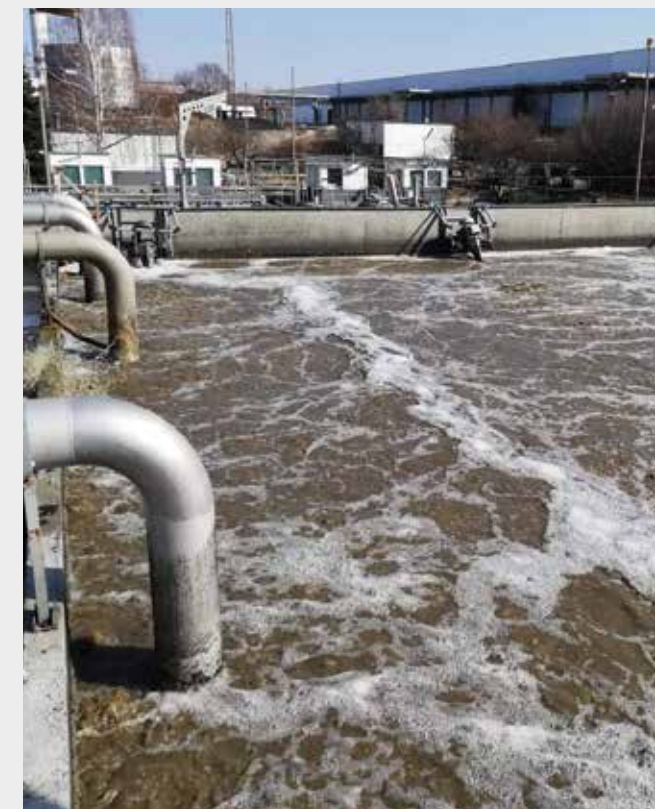
FUCHS Aerators easily supplement the existing compressed air aeration (Bulgaria)
