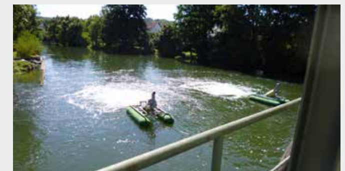
FUCHS Aerators in an emergency application in a river (Germany)
