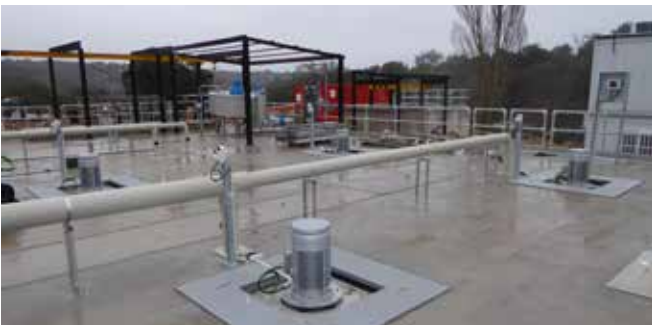
FUCHS Centrox Aerators with foam control for Aerobic Digestion (Spain)
