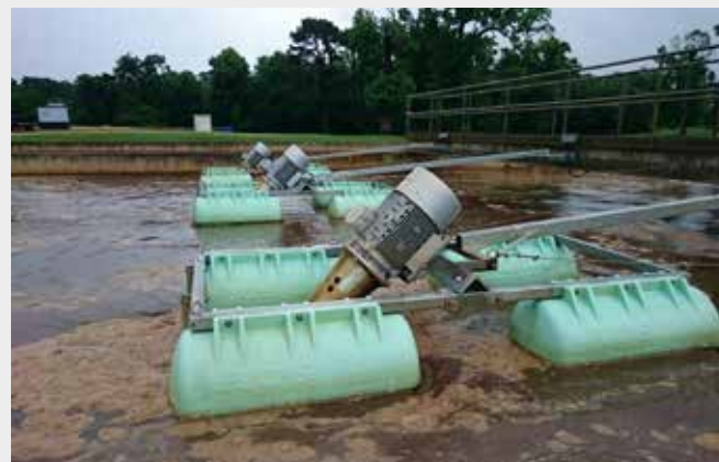
FUCHS Aerators successfully replace old floating brush aerators (USA)
