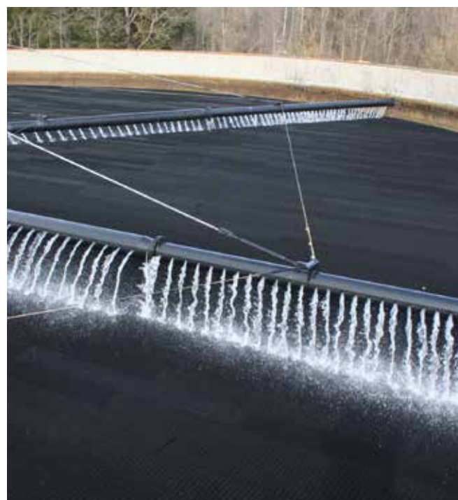
Trickling filters convince with energy efficiency
