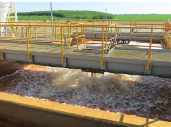
AeroStar Aerators for desorption of CO 2 in mine water (Germany)
