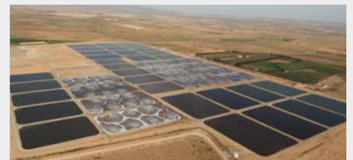
Large aerated wastewater lagoon system with FUCHS Aerators (Morocco)
