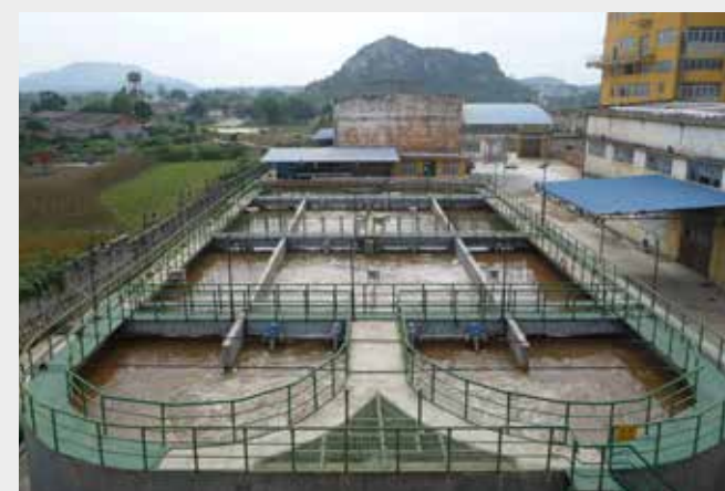
FUCHS Aerators in the activated sludge tank of a sugar factory (China)
