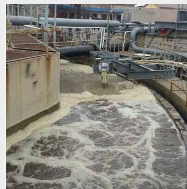
FUCHS Aerators for aeration and mixing of wastewater from textile industry (China)
