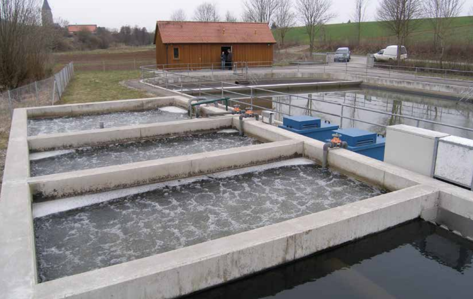
FUCHS fixed-bed system for carbon removal and nitrification (Germany)
