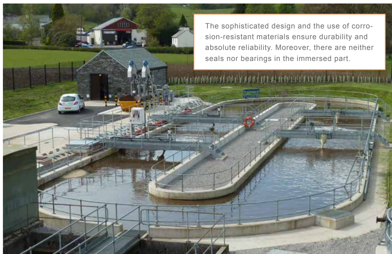
FUCHS Aerators in the oxidation ditch of a municipal WWTP (UK)
