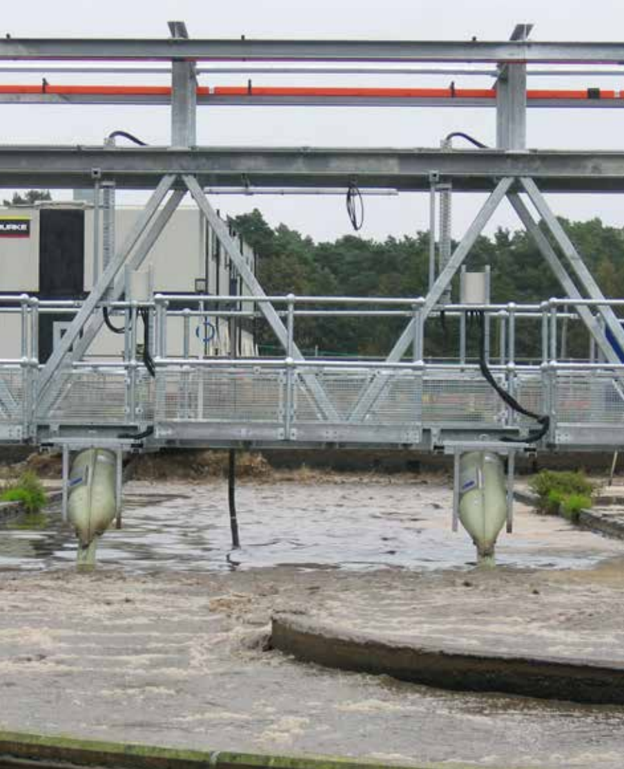
Supplemental aeration in an oxidation ditch (UK)
