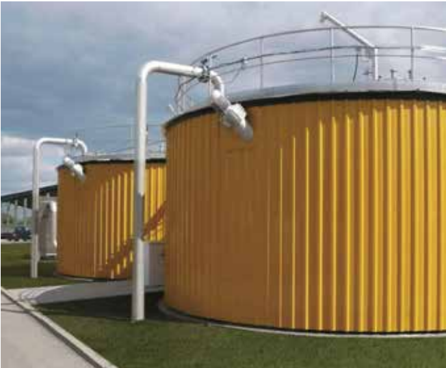
FUCHS ATAD plant for municipal or industrial sewage sludge treatment (Poland)
