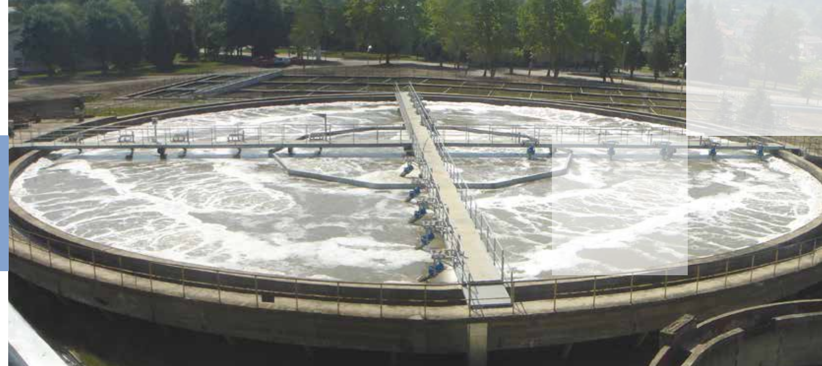
Treatment of paper mill effluent with FUCHS Aerators (Bosnia Herzegovina)
