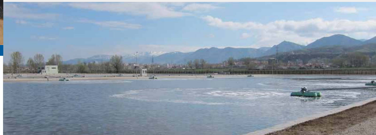
Aerated wastewater lagoon system for 70,000 p.e. (Albania)
