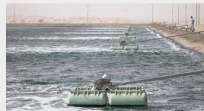
Effective oxygen transfer with FUCHS Oxystar® Aerators (Algeria)
