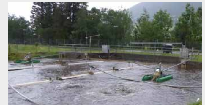
FUCHS rental aerators to compensate an oxygen deficit (Germany)
