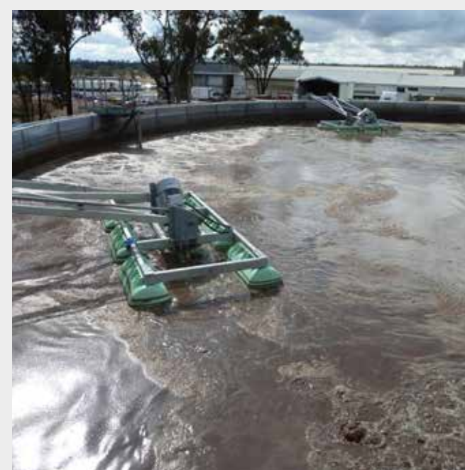
Floating FUCHS Aerators in an activated sludge tank of a slaughterhouse (Australia)
