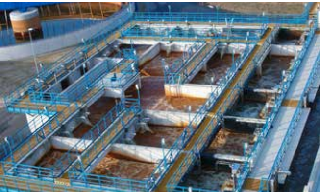
OxyStar® Aerators for oxidation of mine water (Germany)
