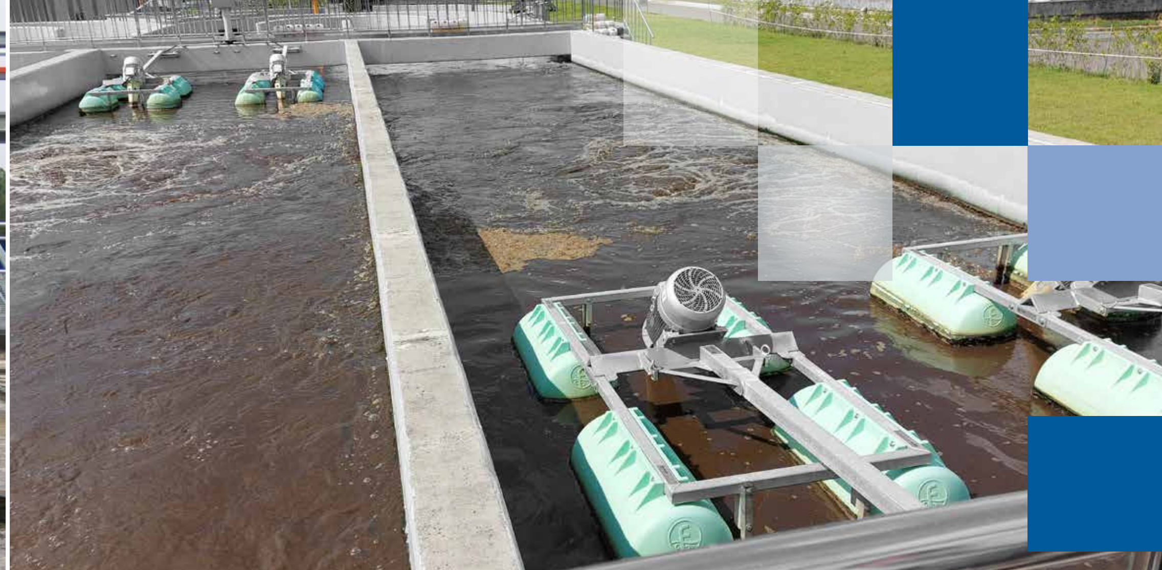
Replacement of brush aerators in municipal WWTP (South Korea)
