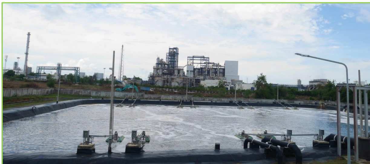
FUCHS OxyStar Aerators in the 2011 newly built equalization lagoon
