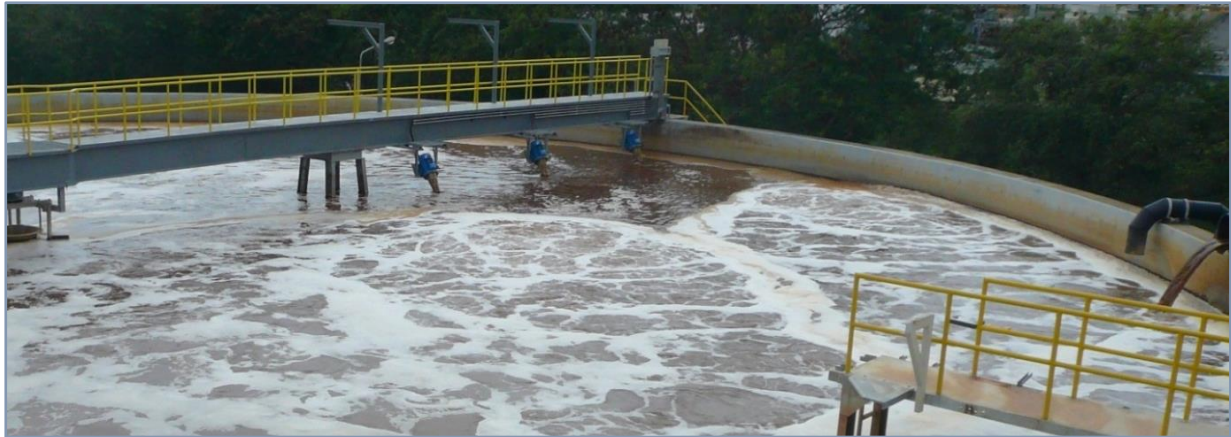
OxyStar Aerators in the new aeration tank (converted former EQ-tank) after expansion in 2006
