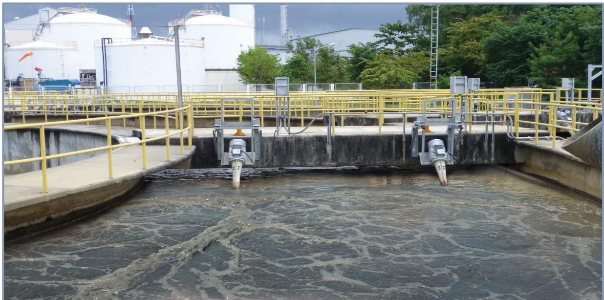
Surface Aerators replaced by OxyStar Aerators in one of the double concentric aeration tanks
