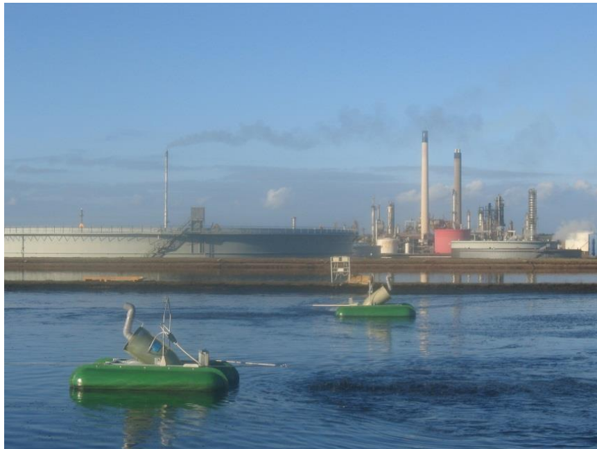
FUCHS OxyStar Aerators in a large lagoon system
