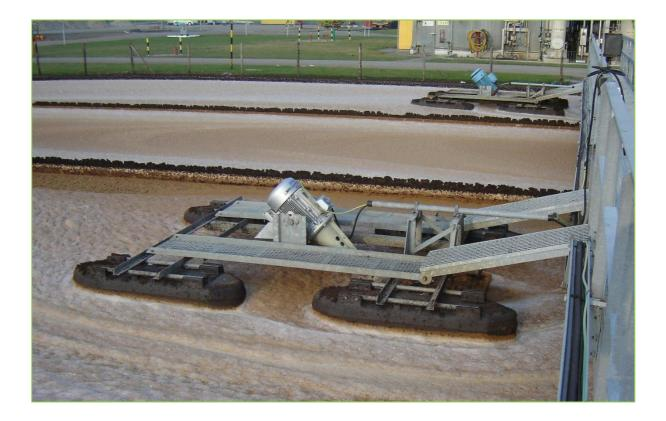
In 2010 a US-based international chemical company needed new aerators to retrofit one of their European wastewater treatment plants. They intended to replace worn US-made aspirating aerators.
