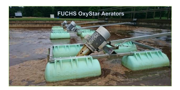
Nine FUCHS OxyStar Aerators type OS 30.0 on flotations were installed at the existing bridges and were fully operational in January 2015. At that time the existing bar screen was also replaced by a new perforated plate filter screen with washer and compactor.
