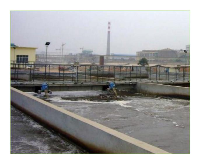
At the end of 2007 the carrousel shaped oxidation ditch of Funan sugar mill was equipped with 34 sets of OxyStar Aerators OS 30.0 (22.0 kW each). The aeration tank has a total volume of approx. 35,100 m<sup>3</sup>.
