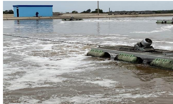
Fig. 4 WWTP El Cortijo: Aeration Lagoon N°2 layout with OxyStar® OS30 aerators in operation in 2022
