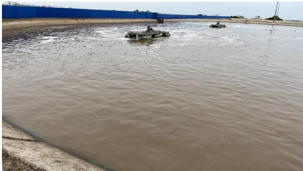
Fig. 4 WWTP El Cortijo: Aeration Lagoon N°2 layout with OxyStar® OS30 aerators in operation in 2022
