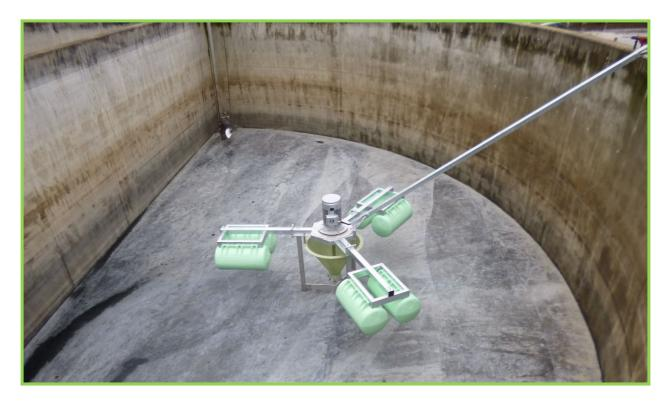
Aerobic Biosolids Digestion with FUCHS CENTROX Aerators is a cost-effective approach for sewage sludge stabilization used at many wwtps in Europe.
