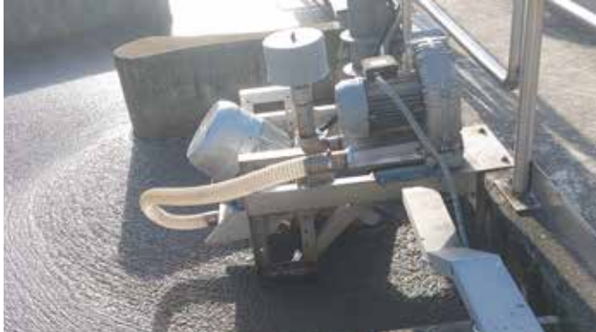
DualStar aerator with mounting bracket on a machine bridge
