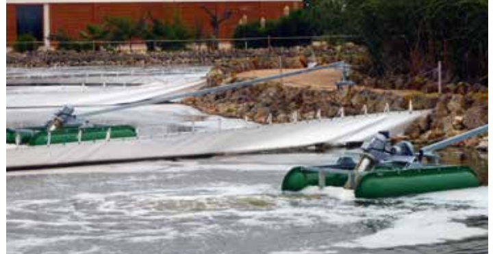
DualStar aerator on floats in a sewage pond system
