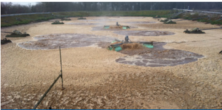
Treatment of wastewater from slaughterhouses and meat processing
