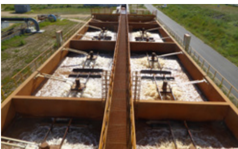
AeroStar aerators for stripping CO 2
