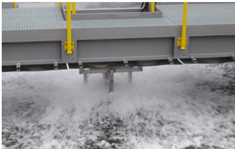
AeroStar aerator with mounting bracket
