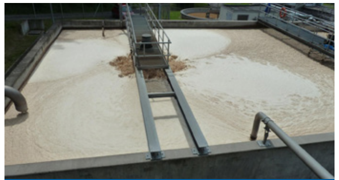
Treatment of wastewater from chemical industry
