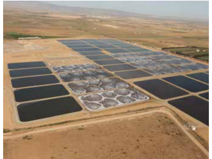
Aerated wastewater lagoon system with OxyStar® aerators (Morocco)
