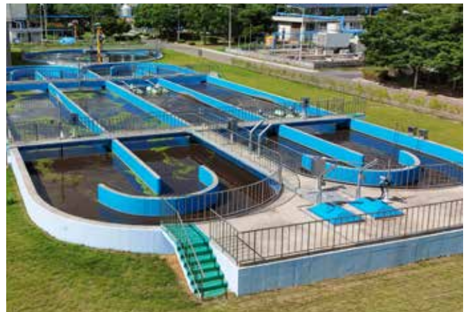
Oxidation ditch of a municipal WWTP (Korea)
