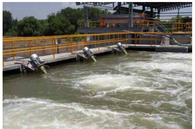
A special application of OxyStar® aerators is the ferrous iron oxidation of mine water
