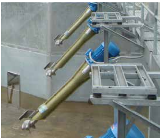
OxyStar® aerator with standard mounting bracket
