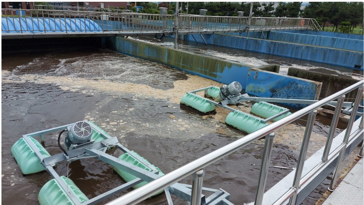
Decommissioned brush aerators (right) and new OxyStar® Aerators (left)!
