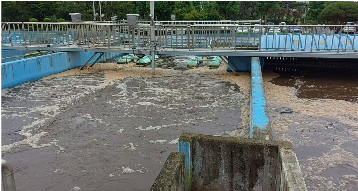
Decommissioned brush aerators (right) and new OxyStar® Aerators (left)!
