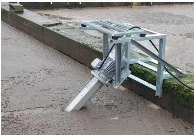
TurboStar® mixer on standard mounting bracket
