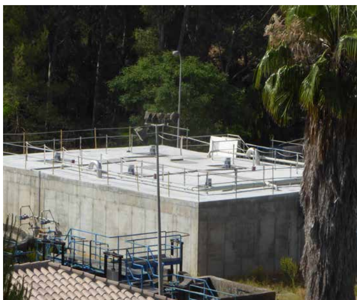
Increasing the performance of a municipal wastewater treatment plant (Spain)
